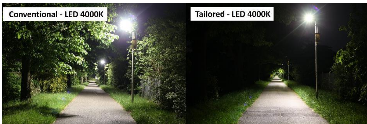
Fig. 2: View of the road illumination (same site as in Fig 1) comparing a conventional LED luminaire (left) to our newly developed tailored and shielded LED luminaire (right). (Images: A. Jechow)
