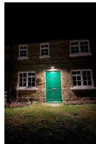
Fig. 1: Hawnby Village scheme – the first complete village retrofit scheme
