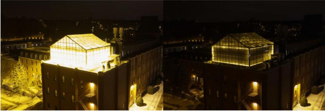
Fig. 2: Comparison of using blackout curtain to limit artificial light from escaping a research greenhouse at Bishop's University in Sherbrooke, Qc. Same exposure settings were used for both images. Photo by Guillaume Poulin / MMISDR
