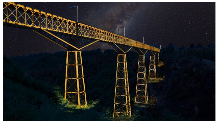
Fig. 5: Malleco Bridge. 800 lighting sources RGA of 8° pointing down and programmed to tell the story of the construction. DIAV by V. Urra.
